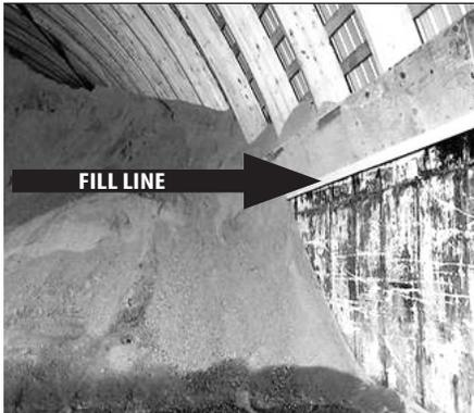
Sand and salt has been filled past the fill point and against walls potentially causing corrosion of connection points and wall displacement.
