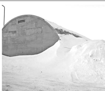
Snow has been allowed to accumulate on the sides restricting ability for snow to shed from the roof and potentially compromising structural integrity.
